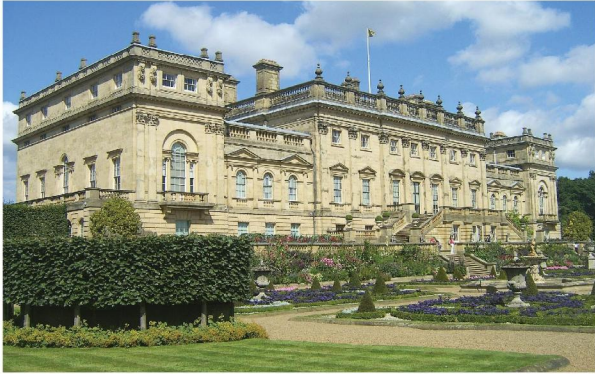
Harewood House, West Yorkshire
