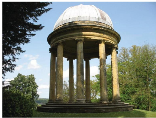
Duncombe Park Ionic Rotunda, North Yorkshire
