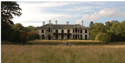
View of the existing house looking north west
